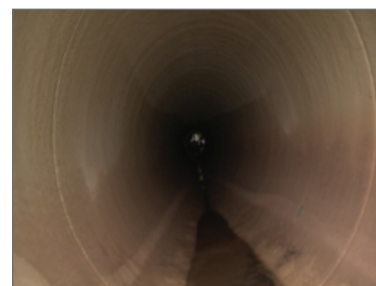
Completed liner at one year inspection.
