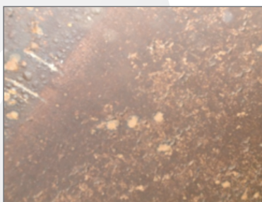
Prepped pipe wall substrate.
