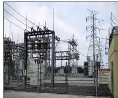
Post Lining: The completed conduit met all customer requirements for structural design and friction tolerance supporting cable connection to the critical power station.
