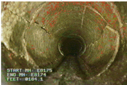
Pre-Rehabilitated Pipeline Condition
